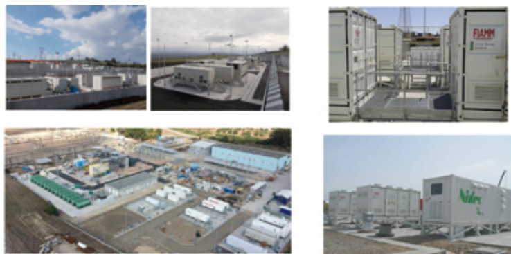
Some photos of Italian large scale stationary electrochemical storage installations
